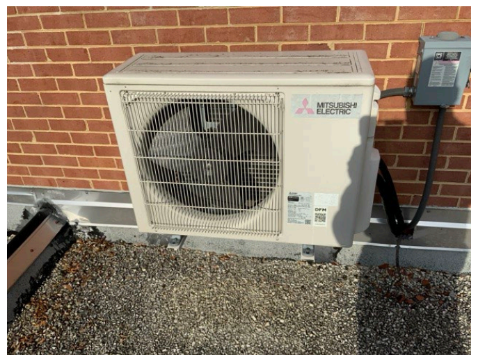
24 - SPLIT SYSTEM DUCTLESS
